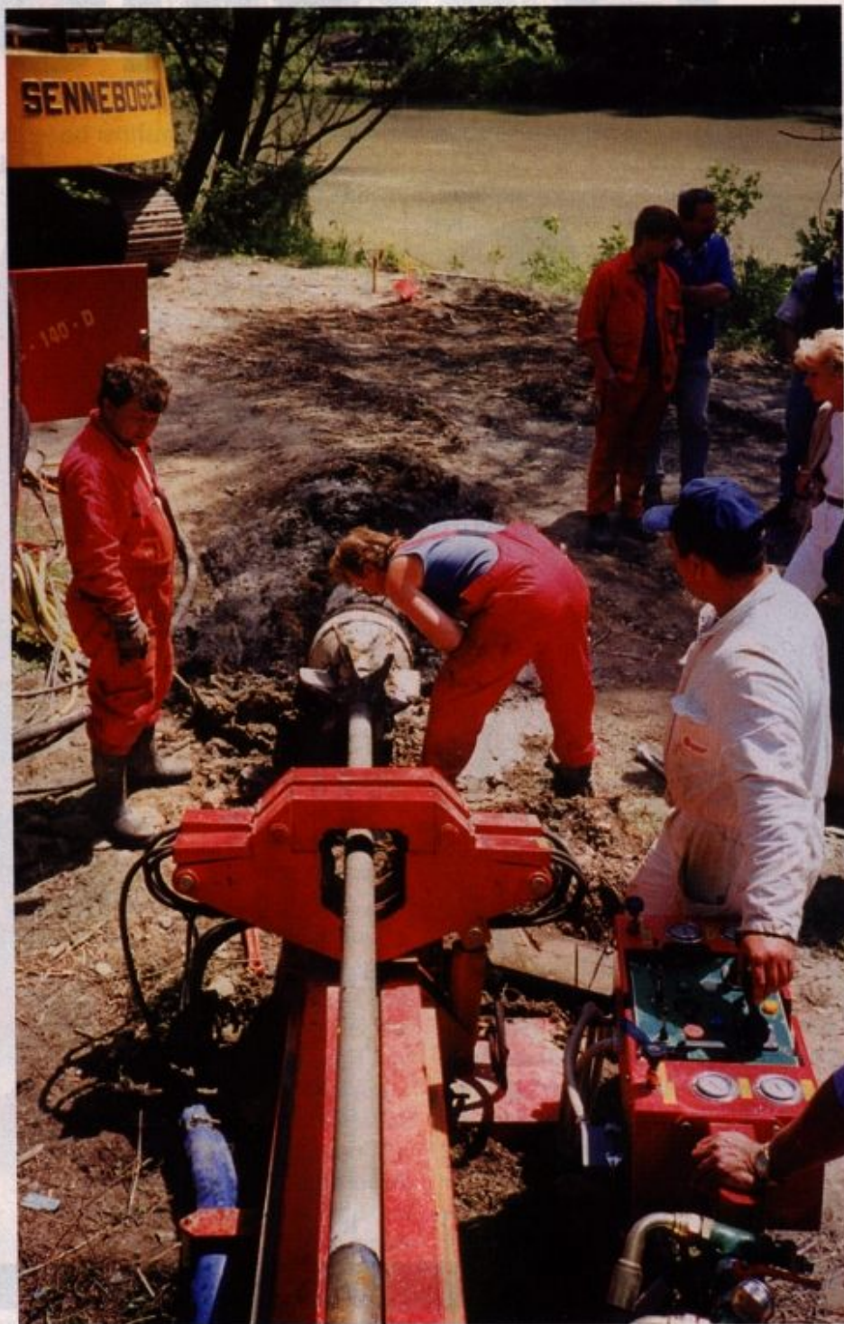
The Scorpio 903 is at its best on downtown jobs, but still able to make small river crossings like this one in Germany.
